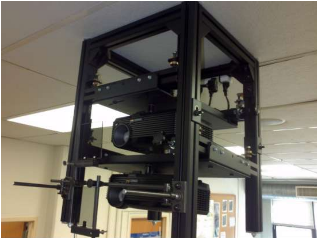
Figure 1. Two small projectors in a ceiling mount.
